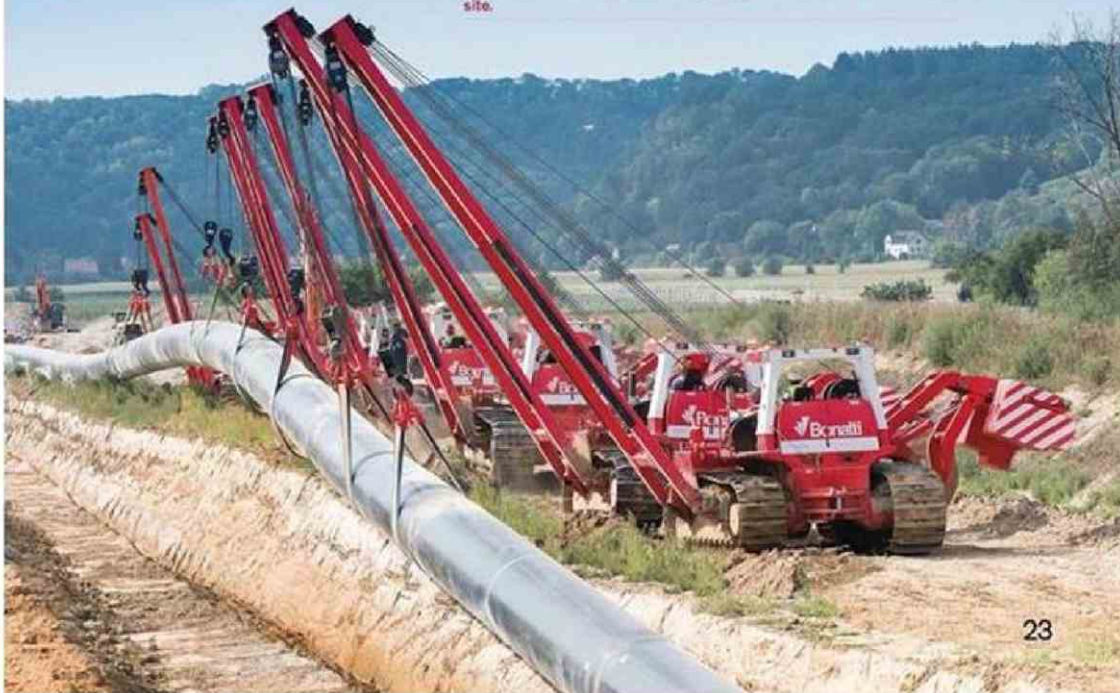
Figure 1. Bonatti Safe-T-Rex 130 pipelayer at work on a construction site.
