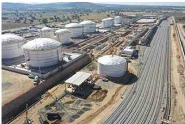
Figure 3. Tank terminal construction, Mexico.
