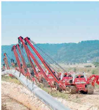
COASTAL GASLINK Bonatti in Canada gestisce 247 km.
